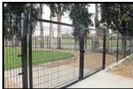
Current typical fence design planned for Duke Energy swim beaches
